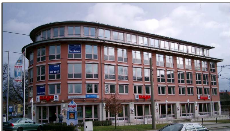
Office and commercial building, Dresden
